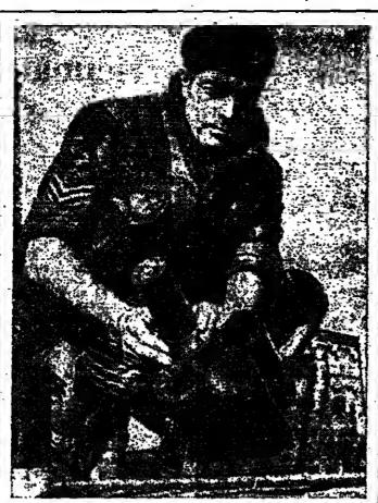
GANG-BUSTER - A British soldier demonstrating new anti-terrorist weapon in Belfast. It is a 4-barrelled launcher for new CS gas grenades which can lay a carpet of gas up to 20 yards wide. Fitted to armored cars, the launcher has a range of about 250 yards and each grenade contains about 400 gas pellets.
